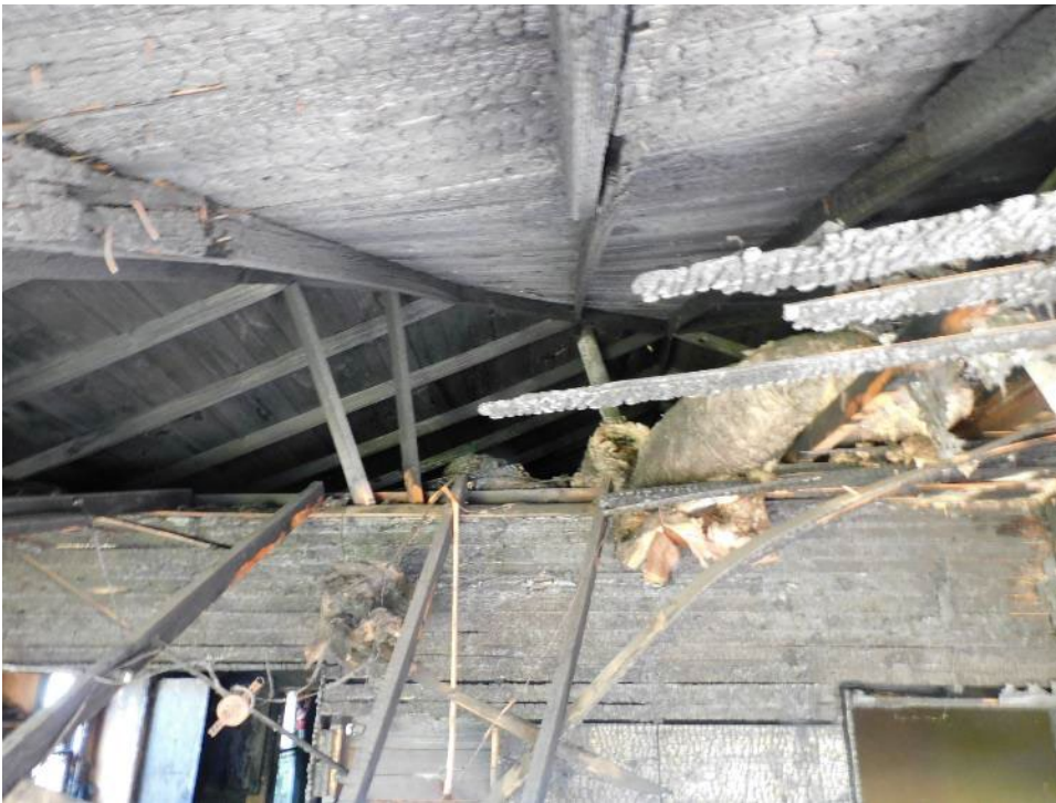
Photo 8, Attic, damaged roof framing.
